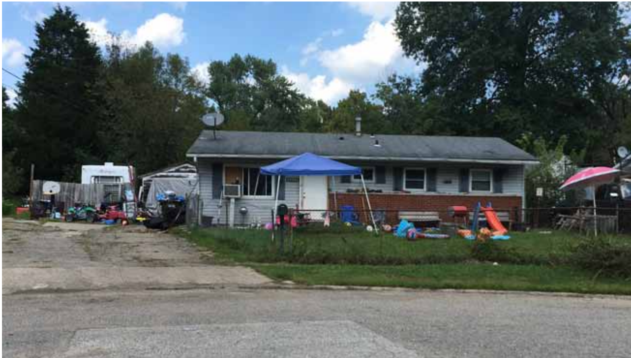
An example of a property maintenance violation
