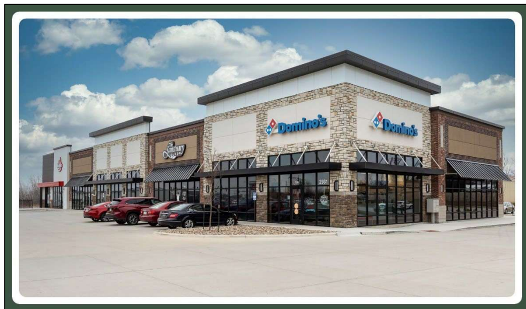
Figure 4.6.2-C - Example Flat Roof with Projecting Cornice
