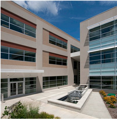
MSD Wastewater Engineering Building
