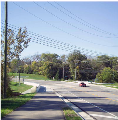
Bethany Road Widening
