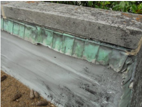
Original copper flashing
