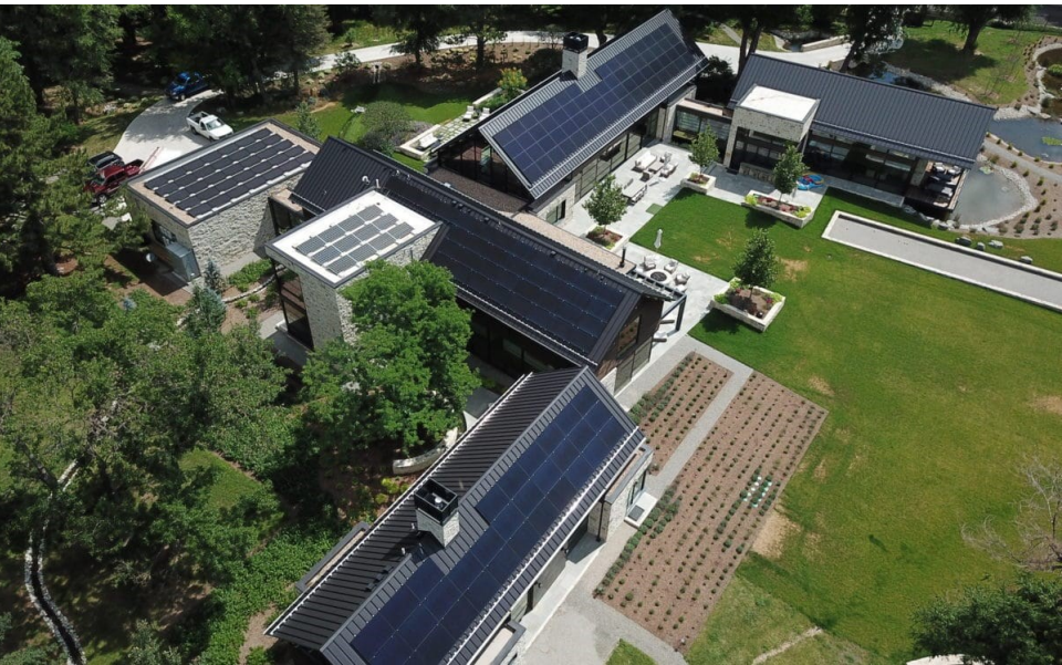
A 10 MW, 40 MWh storage project connected to a community microgrid - Clean Coalition
