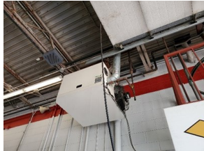
Typ. Gas-Fired Unit Heater
