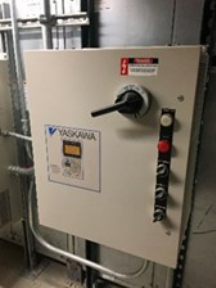
AHU-2 VFD
