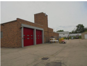
North Bay Doors and Apron
