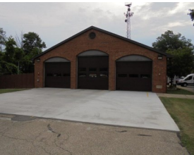
Apparatus Bay Access and Apron
