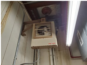
Typ. Electric Unit Heater
