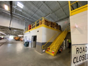
Access to Storage Mezzanine
