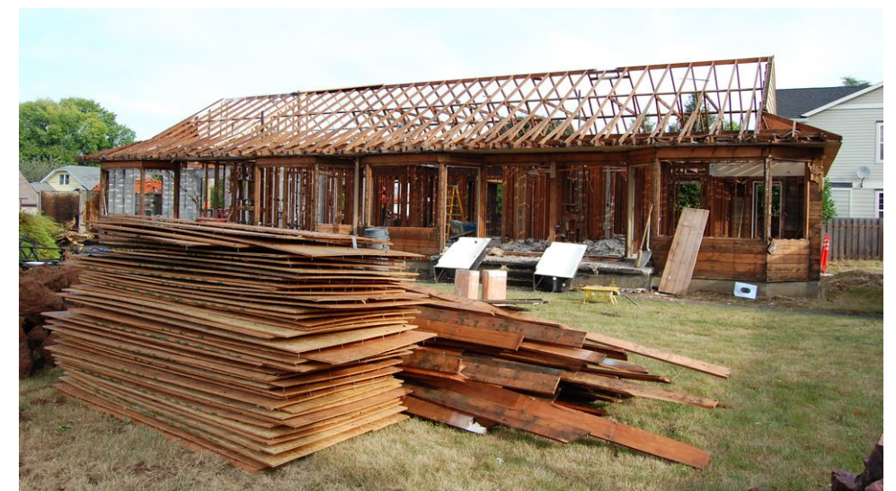
Residential deconstruction / salvage project - ReBuilding Center
