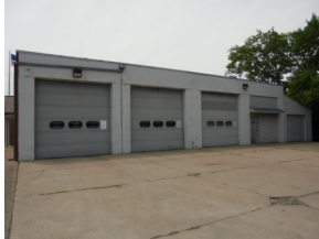
Apparatus Bay Addition
