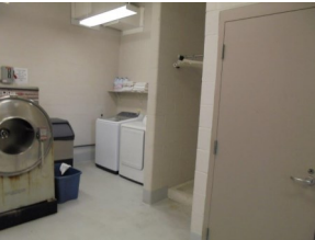
Appropriate Decon Room
