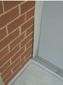
Minor Exterior Repairs
