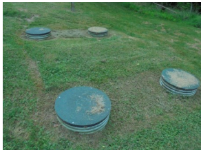
Buried Tank Caps Throughout Site
