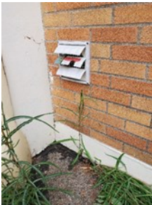
"Flapper" Outlet Damper for Portable AC Unit
