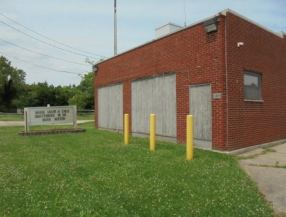
Existing Openings Infilled
