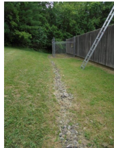
Gravel Drainage Swale
