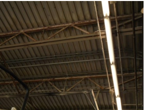
Apparatus Bay Joists
