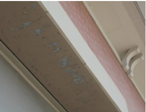
Peeling Paint at Bay Door Lintel
