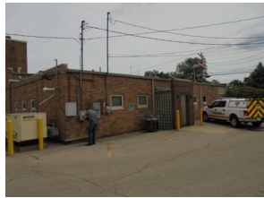
Station 26 Main Entry
