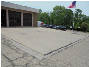
North Bay Doors & Apron
