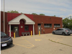
Station 102 Main Entry
