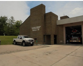
Station 25 Main Entry
