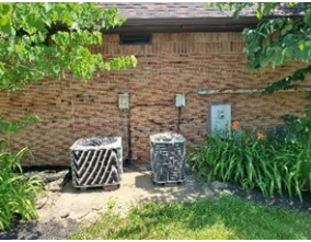
Typ. Condensing Units
