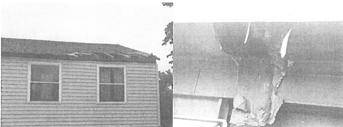
Exterior holes in roof and fascia of the home – EK – 6/17/19
