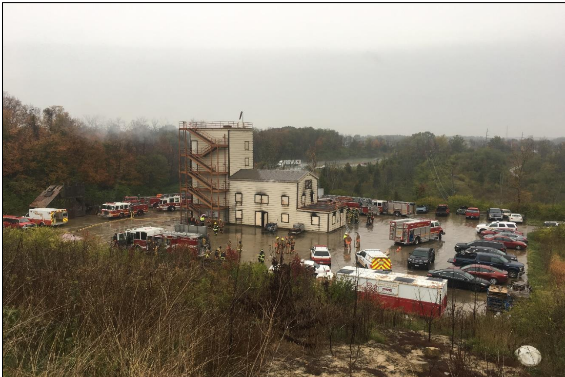
Colerain Township Training Tower: 4200 Springdale Road
